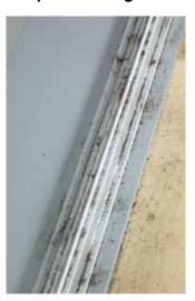
Construction dust, sand grains, hairs from domestic pets, small stones from the garden. Dirt always accumulates, no matter whether during installation or in day to-day use. On the roller, it becomes an unwanted braking mechanism. Gradually it finds its way into the roller. And the unit stops running smoothly. What could be better than simply brushing this dirt away?
