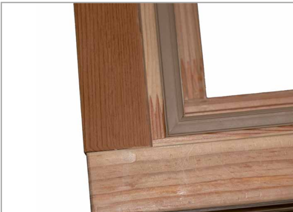
Finished sealing corners
