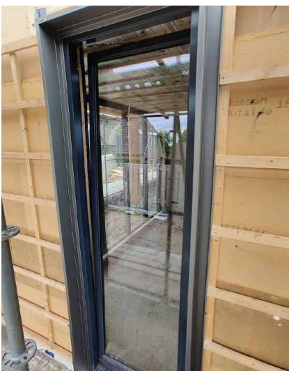
French door with MACO's Multi Power hardware and ventilation scissor stays in large tilt opening (summer position)
